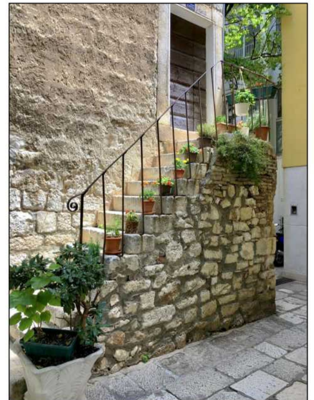
Example - at Crow's Nest natural local stone will be used to match the existing wall, but this photo shows the type of handrail and step configuration to be used.
